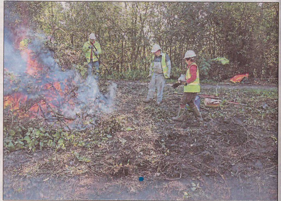
Volunteers carry out restoration work on the Sundorne section in Shrewsbury
