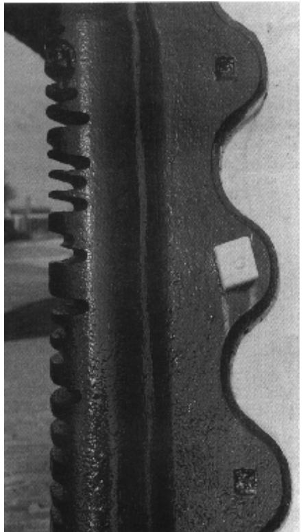
*Where masonry was subject to constant wear from the towropes of thousands of horse-drawn barges, it was reinforced by iron strips which (it is said) still carry the rope scars.*
